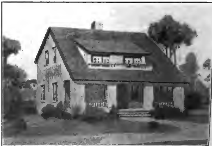
Type of cottage which the Goodyear company is building to furnish its workmen and their families
